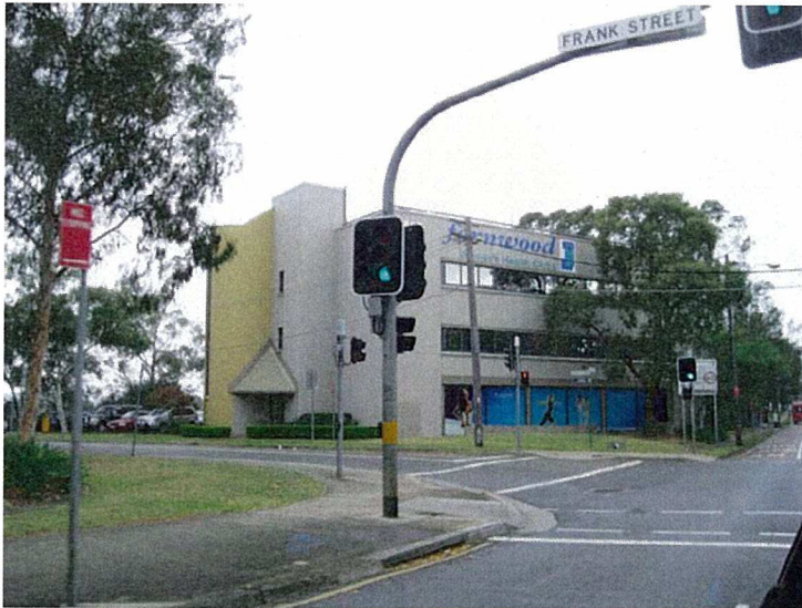
View of 495 Victoria Road – Building H
